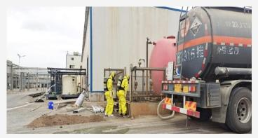
Emergent Closure of the Hydrochloric Acid Storage Tank's Leaking Valve
